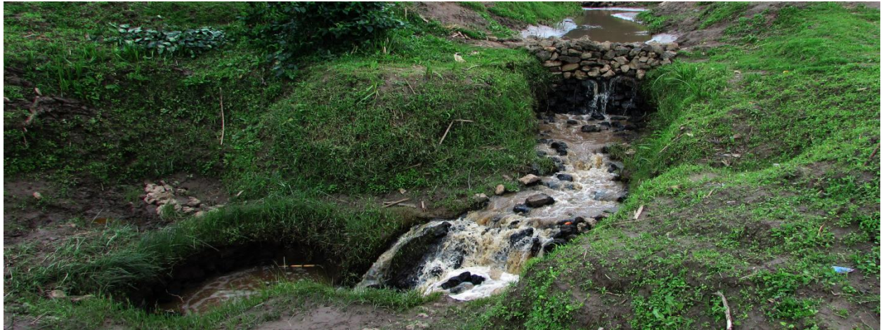
Photo 6: Gabion to retain sediment and a lava pipe where the water flows, Mugogo Valley
